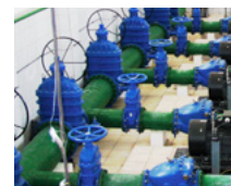
WATER PLANT WORK
